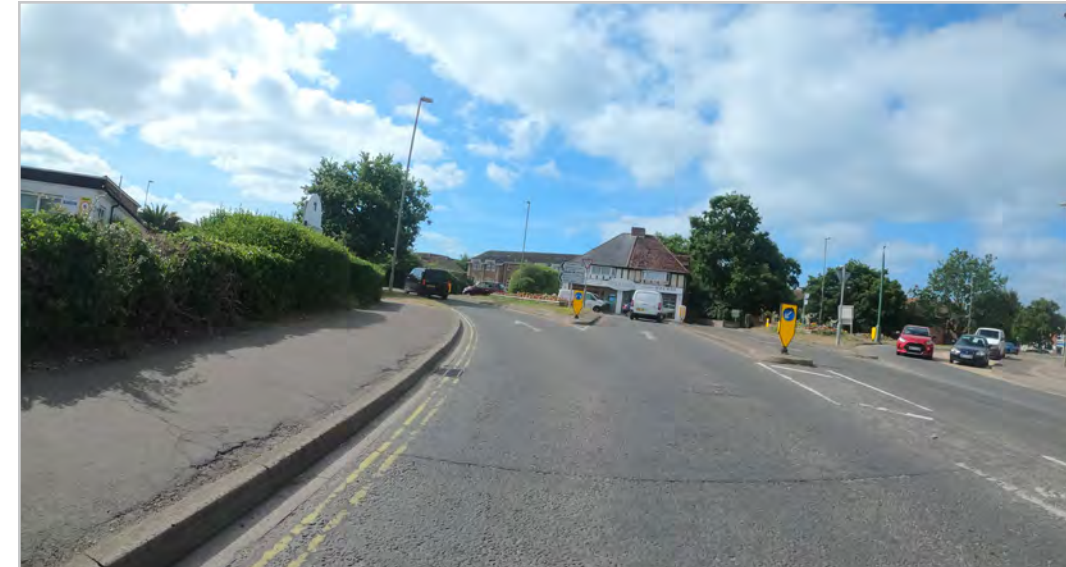
Z3.1.14 – A337/Old Milton Road junction
