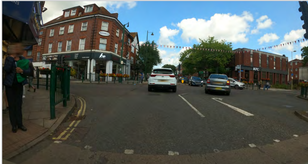
Z3.1.11 – Ashley Road/Old Milton Road junction
