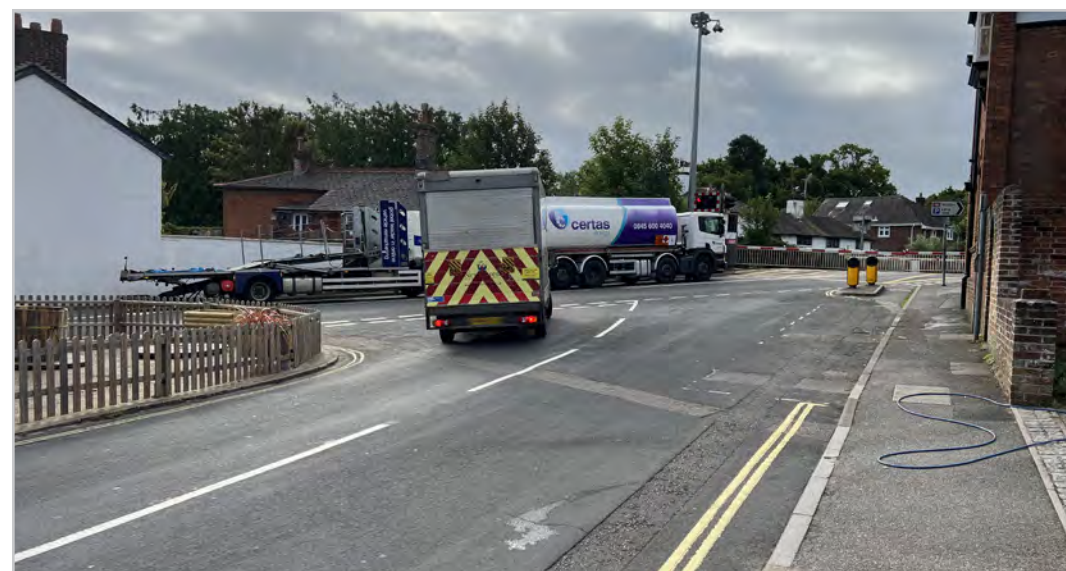
Z6.1.3 – Brookley Road/Lymington Road junction
