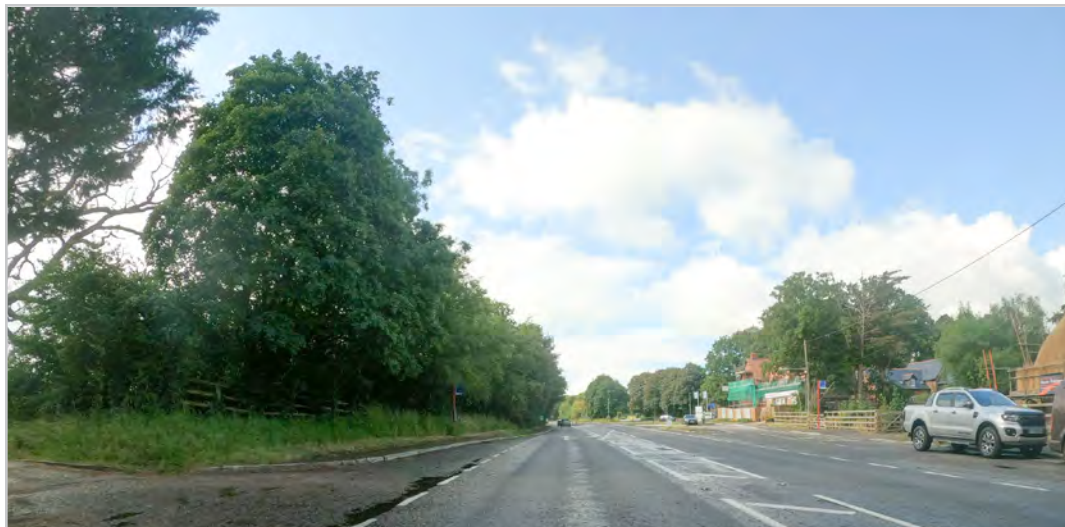
100.1.8 – Salisbury Road between Lower Burgate and the A338/C148 junction
