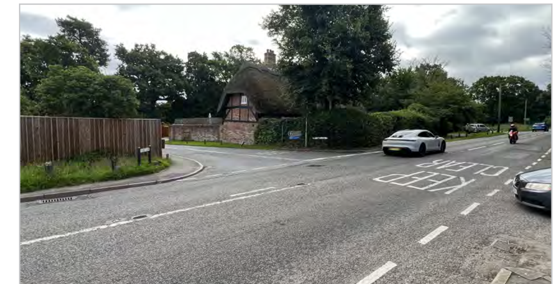
Z6.1.10b – Lymington Road/Mill Lane junction
