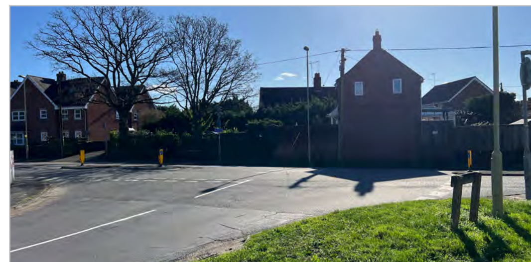
Z2.1.2 – Southampton Road/Gorley Road mini-roundabout
