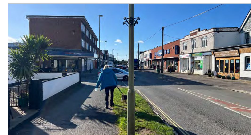
Z3.1.8 – Old Milton Road south of Gore Road
